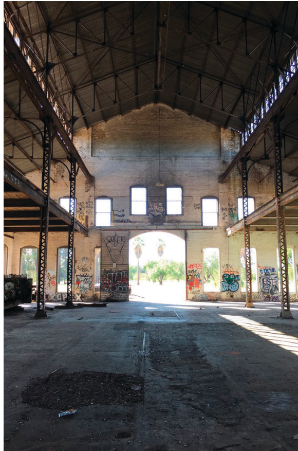
Figure 4.18 Interior view of the existing Engineering Building
