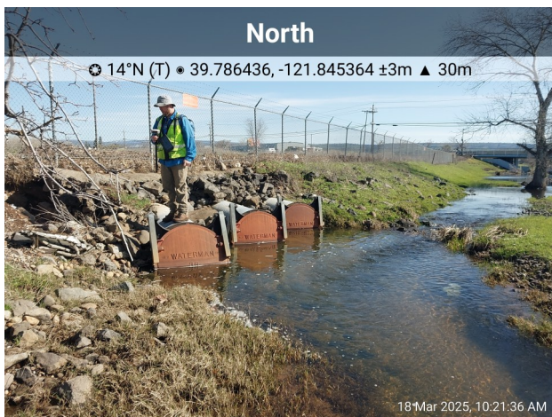
Photo 3. ID-01 View of controlled culverts connecting input flow from ED-03.
