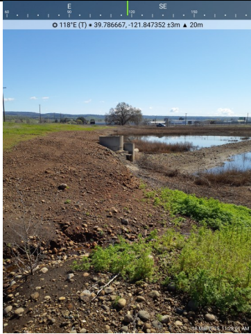
Photo 7: erosional scour from inlet to the stormwater/ wastewater detention basin. Note the dark compost discharge from upslope facility.
