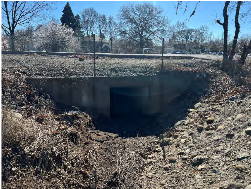
Photo No. 8 SUDAD Ditch culvert beneath Eaton Road
