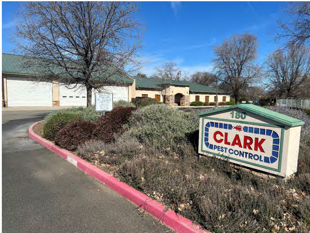
Photo No. 10 Adjacent commercial building at 180 Eaton Road
