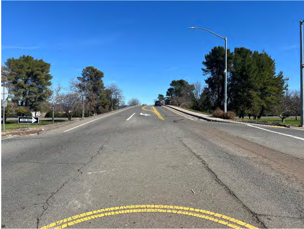
Photo No. 1 Proposed roundabout location west of the SR-99 Eaton Road Overcrossing
