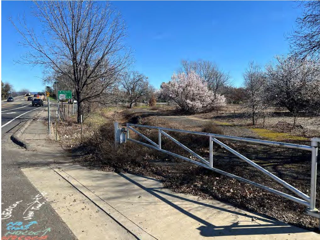
Photo No. 7 SUDAD Ditch south of Eaton Road
