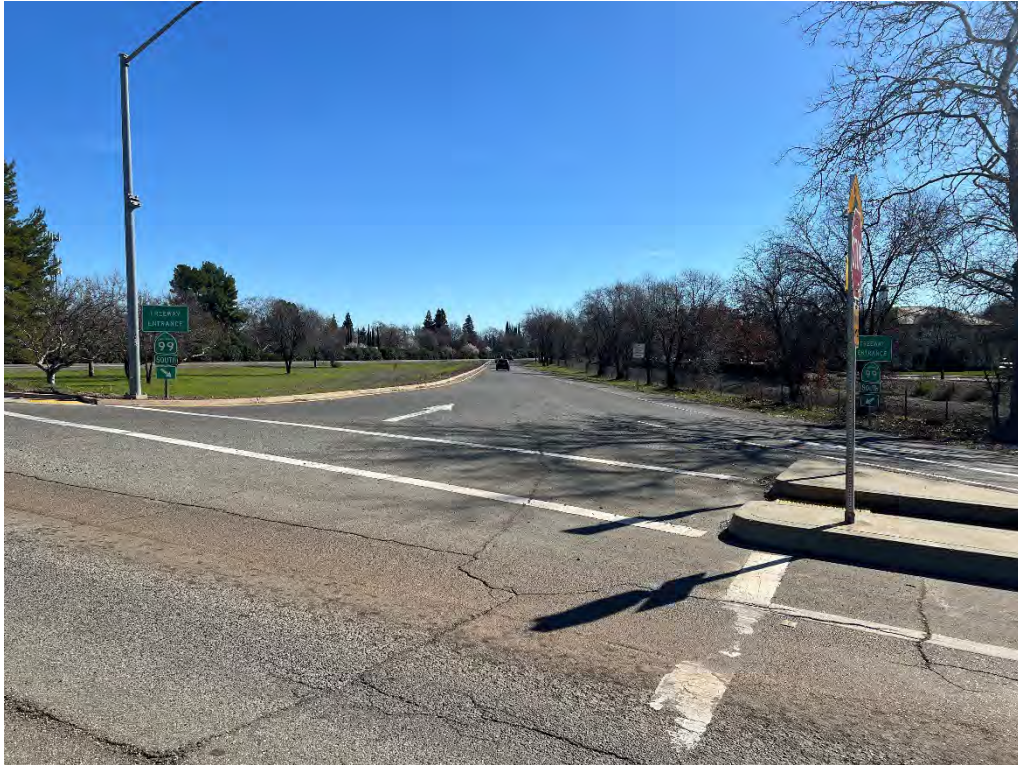
Photo No. 5 Southbound SR-99 On-ramp
