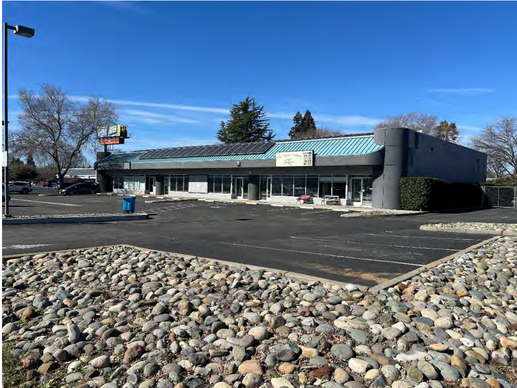
Photo No. 9 Adjacent commercial building at 166 Eaton Road
