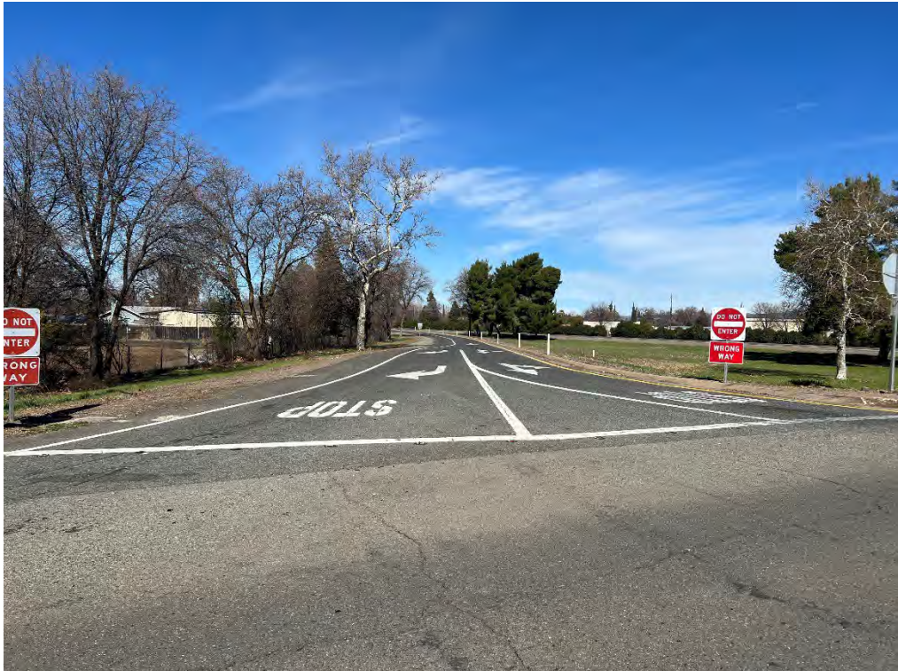
Photo No. 4 Southbound SR-99 Off-ramp
