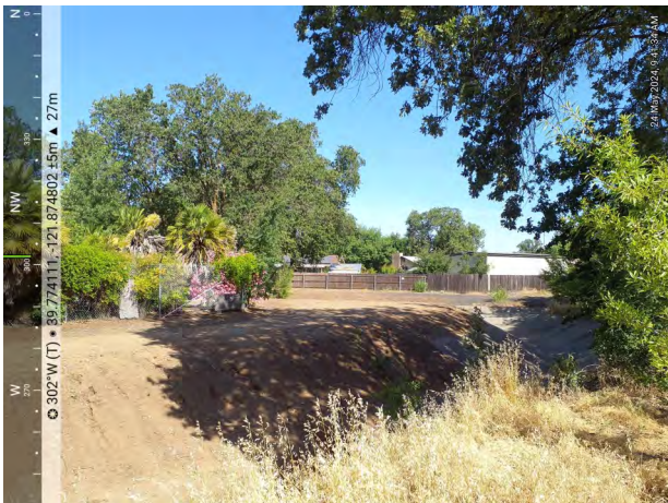
Photo 11. Drainage adjacent to southbound SR99 off-ramp.
