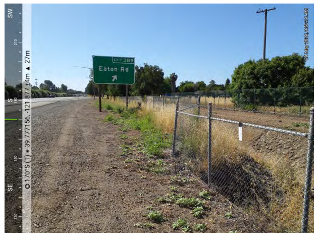
Photo 12. Looking south where drainage turns west and emerges from crossing under SR99.
