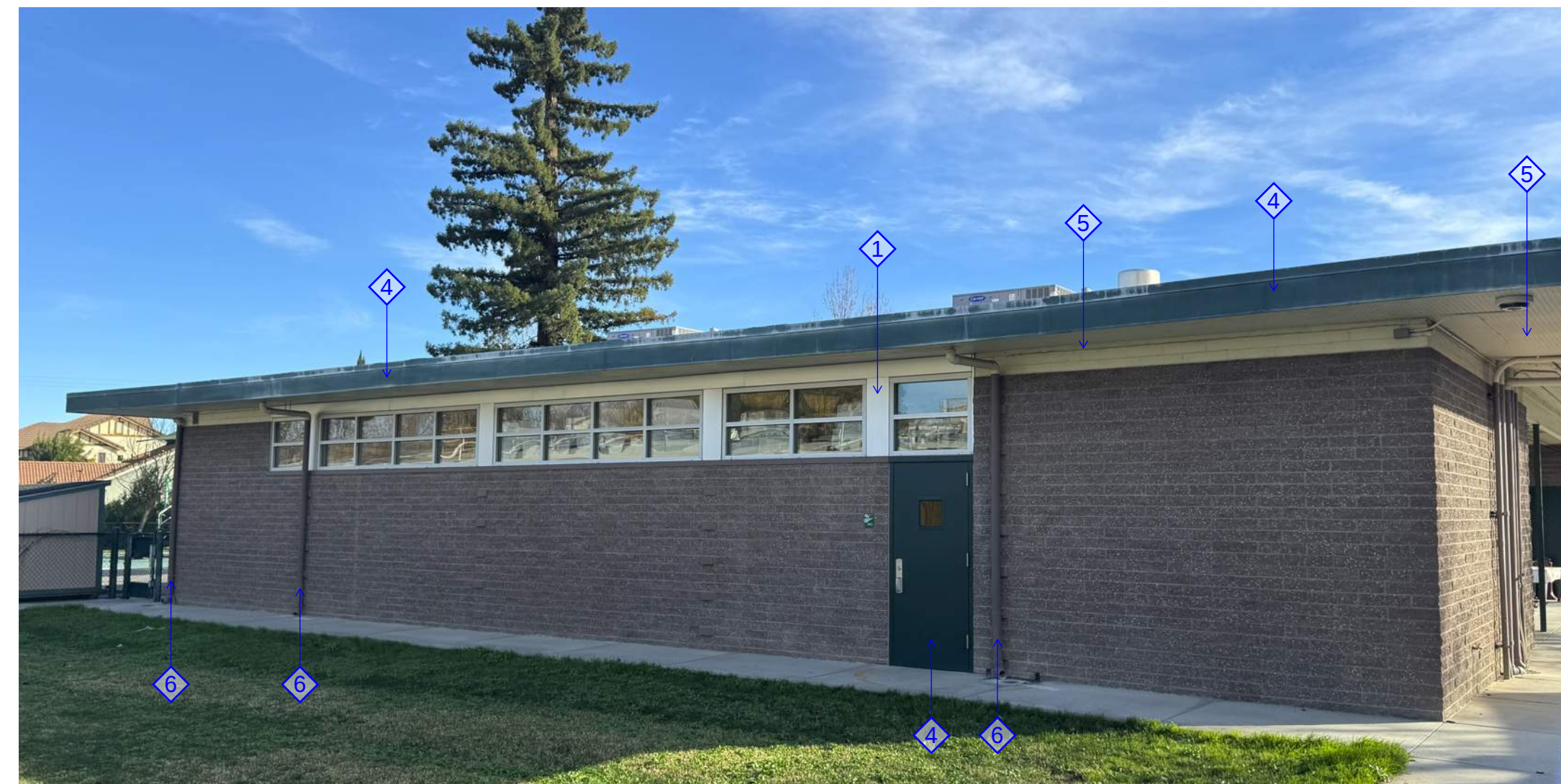
This photograph shows the exterior of a building with a concrete overhang. Several pipes and conduits are visible running along the underside of the overhang. A green support pole is positioned in the foreground. Blue annotations include a line from point 5 to a pipe and a line from point 6 to a wall joint.
