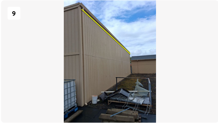
Overall Rear Gutter Line
