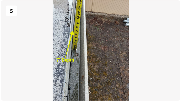
Gutter is 7" In depth
