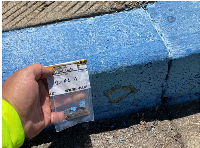
South Parking Lot: View of Sample 2-PC11. The blue paint and underlying red paint on concrete curbs were identified to contain lead-containing paint (LCP) at 1,700 ppm.
