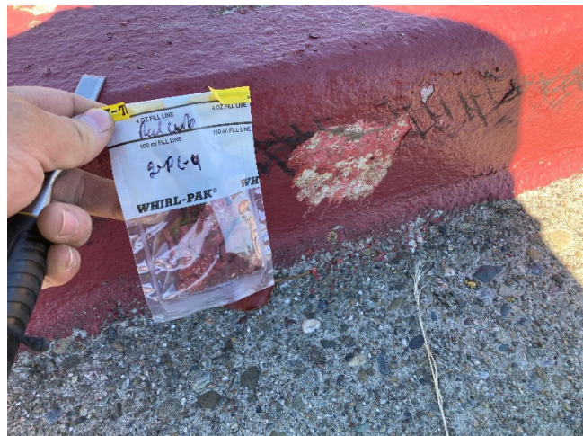
South Parking Lot: View of Sample 2-PC11. The blue paint and underlying red paint on concrete curbs were identified to contain lead-containing paint (LCP) at 1,700 ppm.
