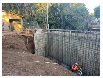
During the month of August, Construction on the north and south bridge abutments was completed opening the door for the contractor to begin construction of the temporary false work required to pour the concrete bridge deck. Prior to construction of false work however, the contractor removed the temporary stream diversion and re-graded the stream channel and installed Rock Slope Protection (RSP) along both stream banks.
