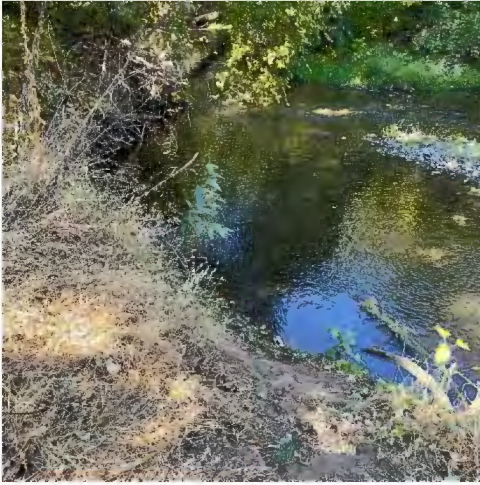
Figure 5: Site 3 Erosion and Characteristics (Looking downstream)
