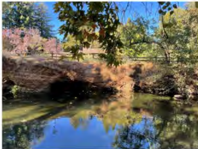
Figure 11: Site 8 Erosion and Characteristics (Looking perpendicular)
