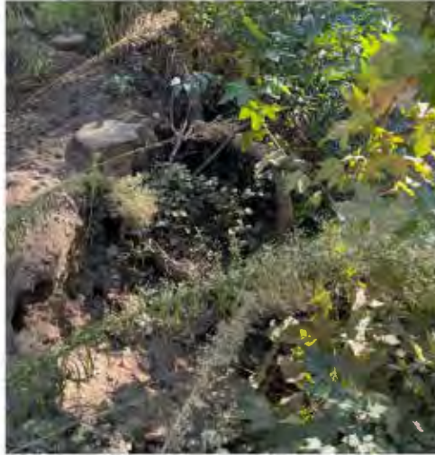
Figure 10: Site 7 Erosion and Characteristics (Looking upstream)
