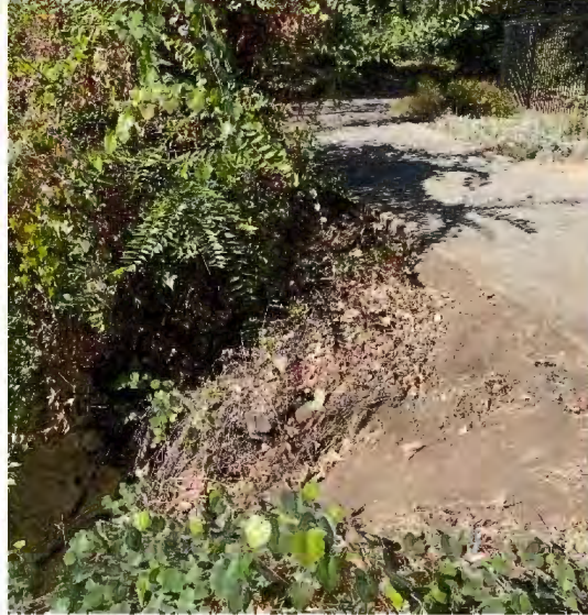
Figure 12: Site 9 Erosion and Characteristics (Looking downstream)
