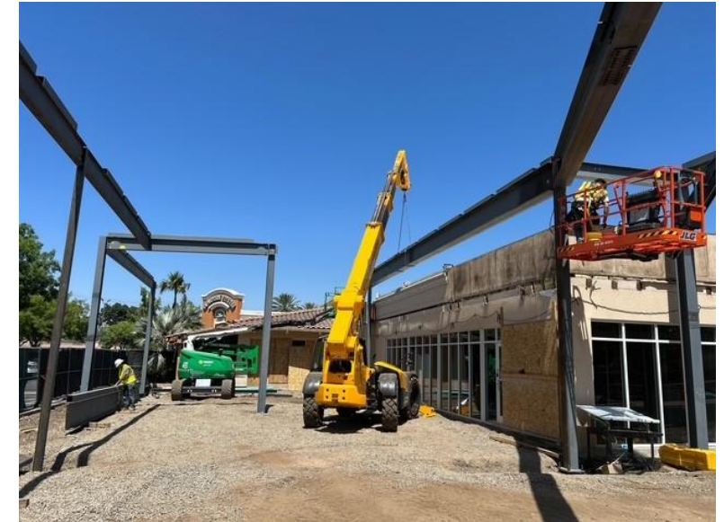
In Motion Fitness Construction Photo Credit: Holt Construction
