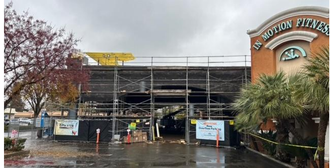
In Motion Fitness Construction Photo Credit: Holt Construction
