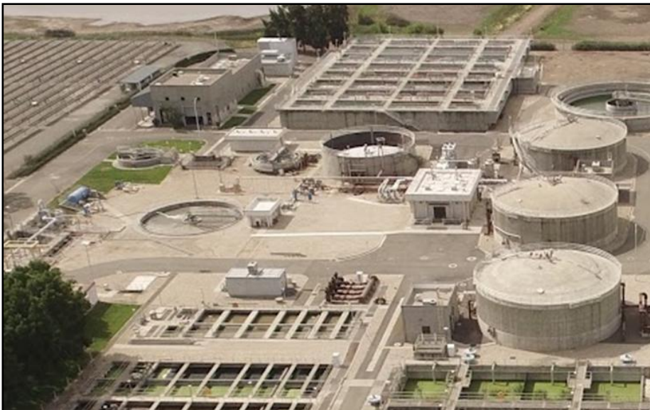
Water Pollution Control Plant
