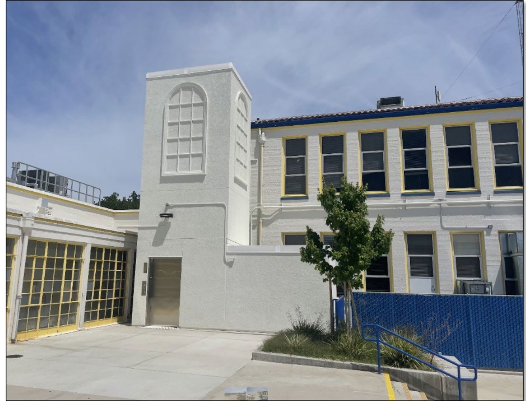
Grant High School Elevator Addition
