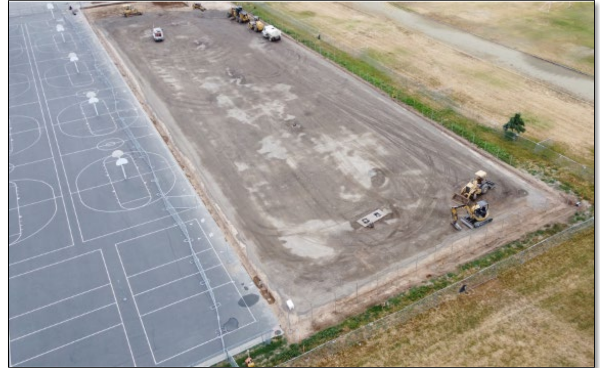
Martin L. King, Jr. Tech Academy (in progress)
