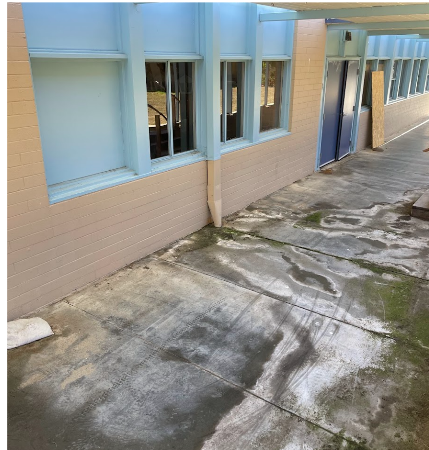
Library basement flooding remediation Damage appears to be from single rain water leader at sunken courtyard
