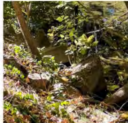
Figure 4: Site 2 Concrete Blocks (Looking downstream)
