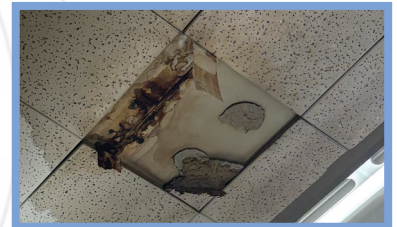
Deteriorating ceiling due to leaking roof at Cavitt Junior High School
