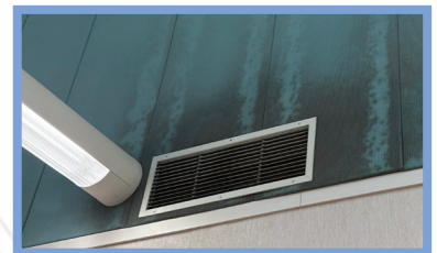
Moldy AC vent at Oakhills Elementary School
