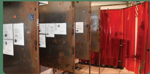
Outdated facilities in classrooms
