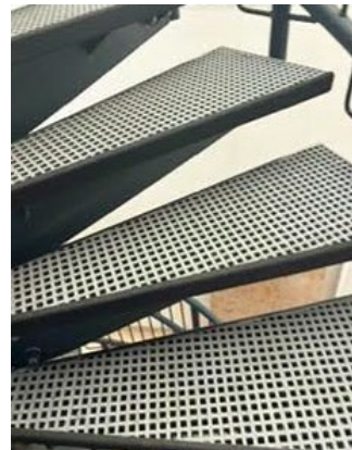
Pool Stairs After
