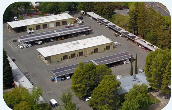
Solar Arrays at Municipal Service Center
