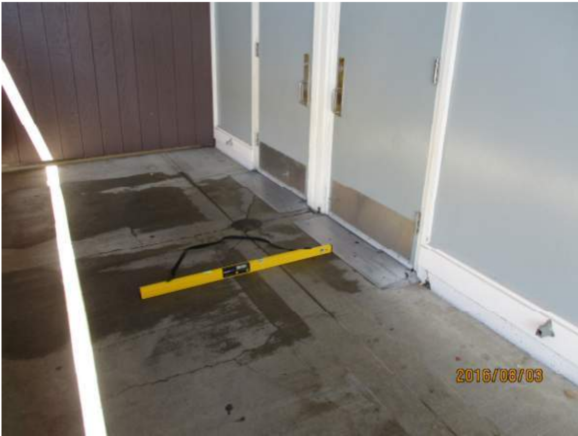
MOUNTAIN VIEW HIGH SCHOOL NON-COMPLIANT THRESHOLD AND LANDING
