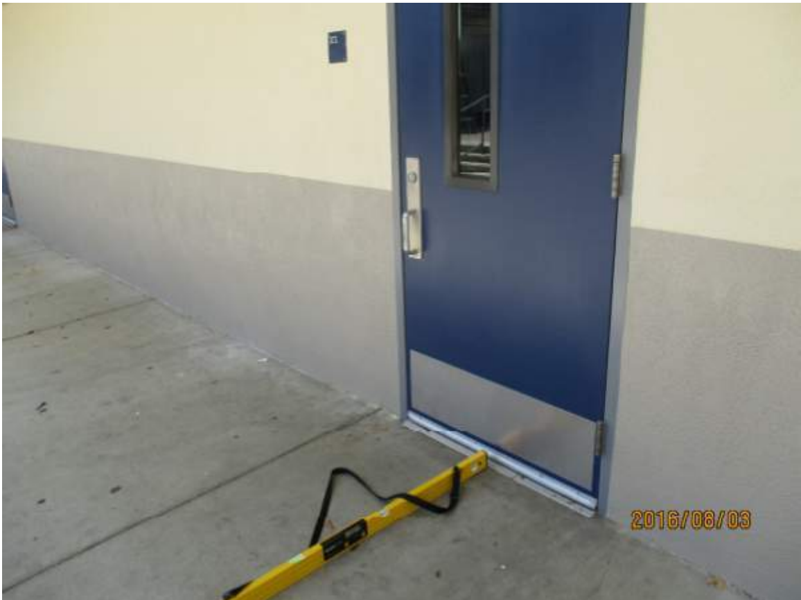
LOS ALTOS HIGH SCHOOL LANDINGS WITH SLOPES GREATER THAN 2%
