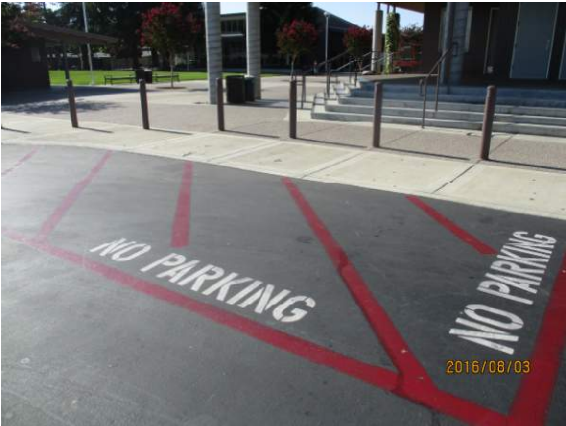
MOUNTAIN VIEW HIGH SCHOOL MISSING TRUNCATED DOMES AT WALKOUT
