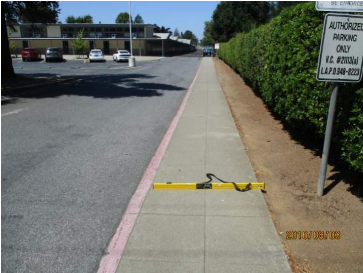
LOS ALTOS HIGH SCHOOL CROSS SLOPE GREATER THAN 2%
