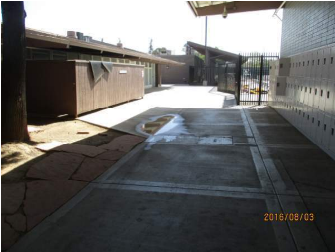
MOUNTAIN VIEW HIGH SCHOOL INADEQUATE DRAINAGE AND PONDING
