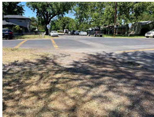
Arbutus Avenue and East 3 rd Street pavement and crossing conditions
