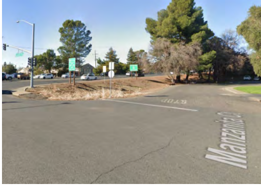
Manzanita Court is a road near SR 99 near an area with pedestrian collisions. It has no sidewalks on one side and limited crosswalks, increasing risk for pedestrians.
