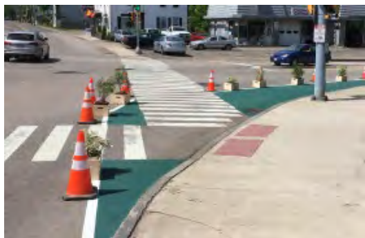
Curb extension in Portsmouth, NH using colorful surface treatments, cones, and plants
