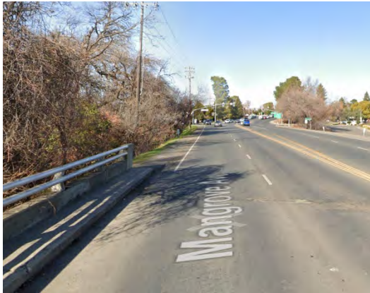
Mangrove Avenue is a State Route where the sidewalk abruptly ends after the bridge. There are also few pedestrian crossings on this segment, increasing pedestrian risk.
