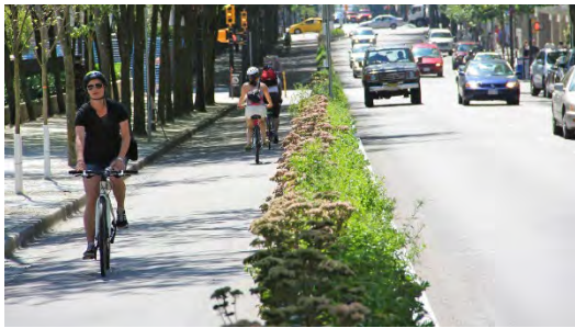
Class IV separated bikeways shield bicyclists from vehicular traffic, increasing safety and comfort for “interested but concerned” riders.
