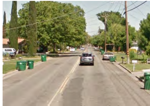
Floral Avenue is a residential street near a high collision density area. The lack of sidewalks increases risk for pedestrians.
