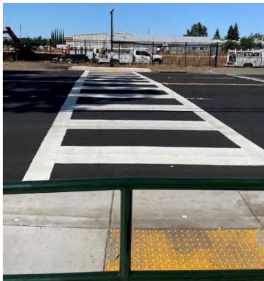
New RRFB crossing on Fair Street in South Chico
