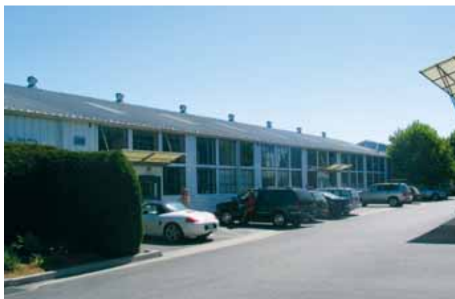
Live/Work housing in Santa Cruz, California.
