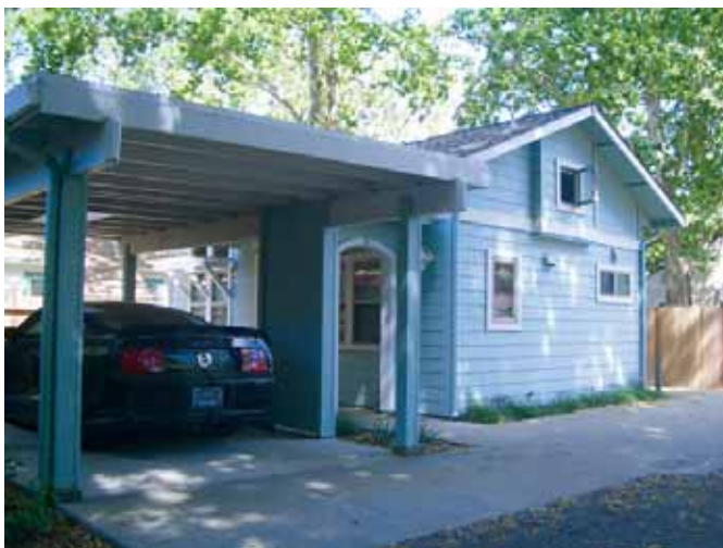
Windows of second dwelling unit facing alley.
