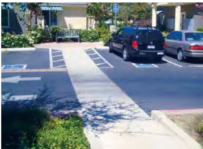
Continuous pedestrian paving identifying clear pedestrian walkway.
