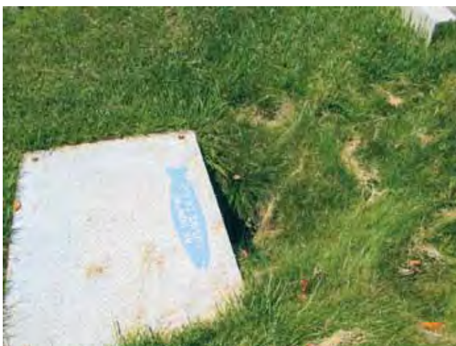
Educational signage on storm drains.
