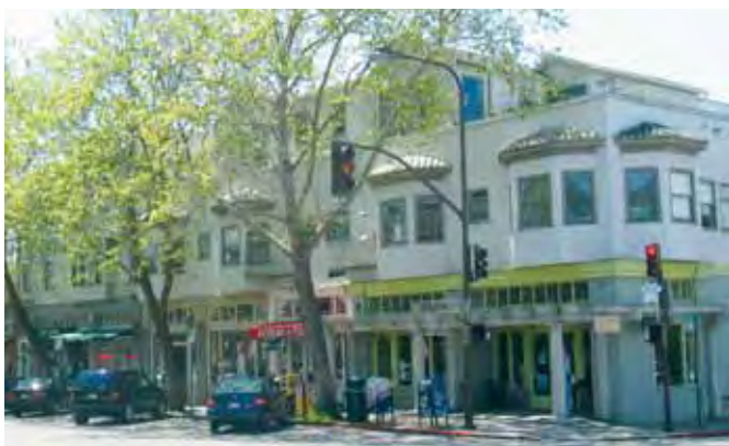
Mixed-use building in Rockridge neighborhood, Oakland, CA.
