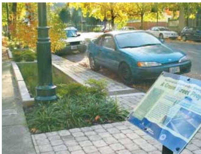
Green Street project in Portland, OR designed to capture street runoff.
