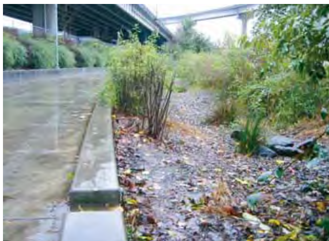
An example of perforated curbs which allow water to infiltrate in a swale.
