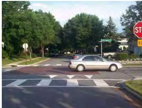
Figure 5-10-J. Speed Platform (Raised Intersection).
