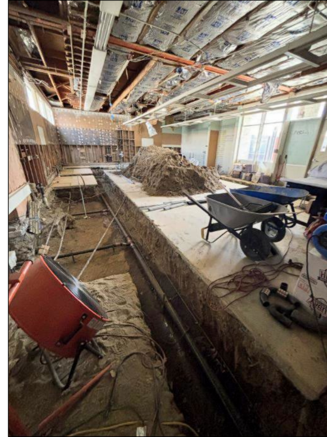
Foothill HS Culinary Classroom Modernization (In Progress)
