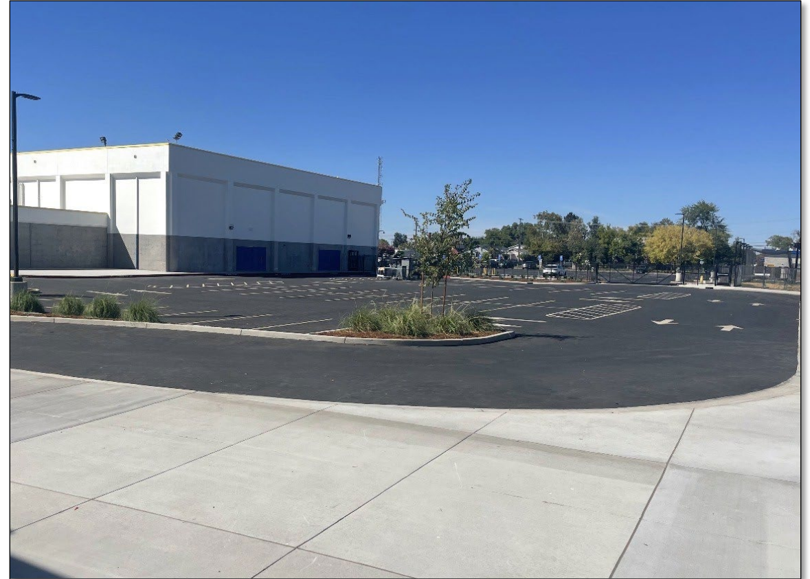
Grant High School Hardcourts Phase 2 (Completed)
