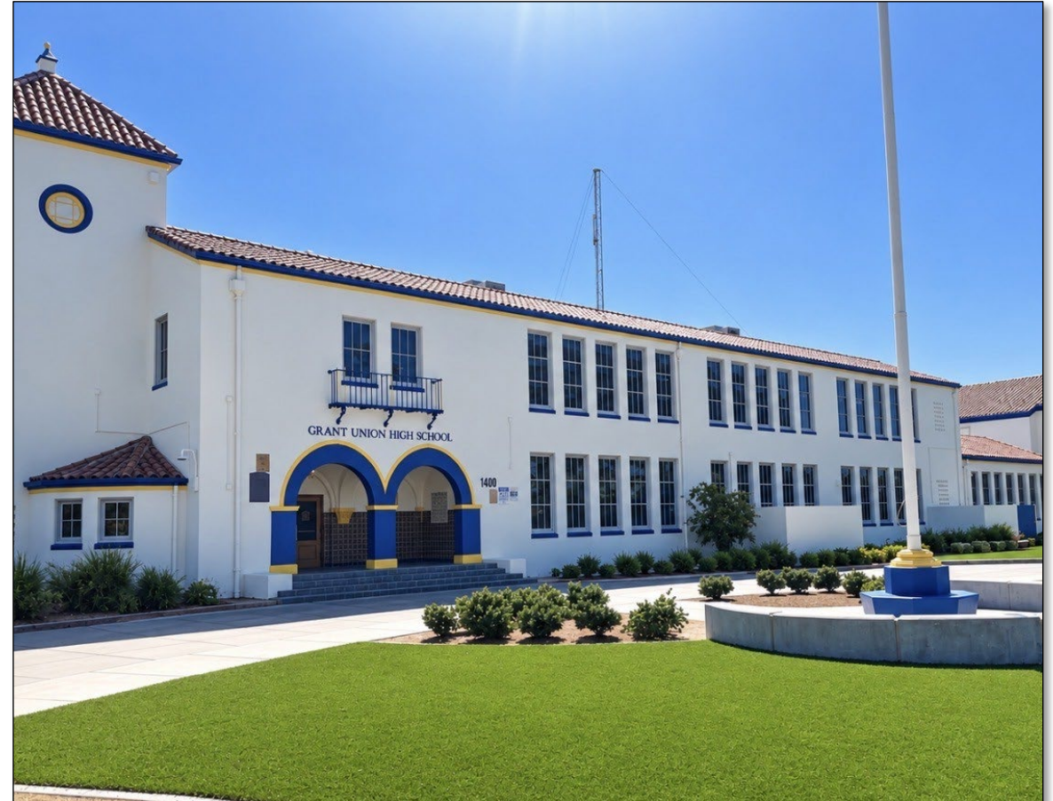
Grant HS Exterior Paint (Completed)
