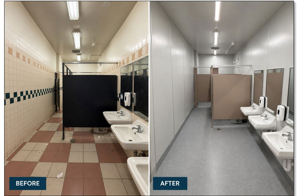
Foothill HS C-wing Girls Restroom
