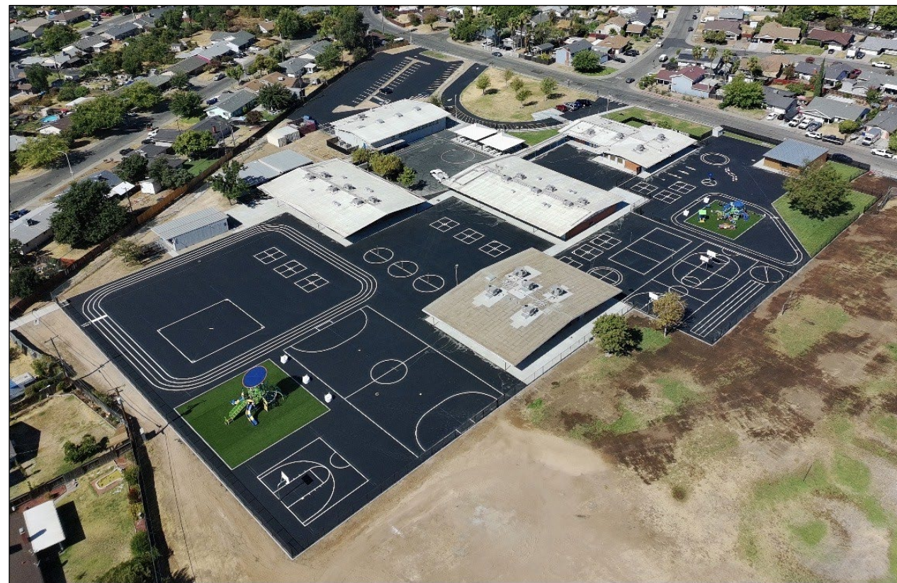
Sierra View ES (Completed)
