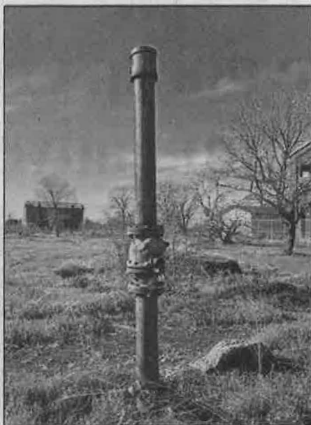
Utilities infrastructure remains at Barber Yard in southwest Chico on Monday.
