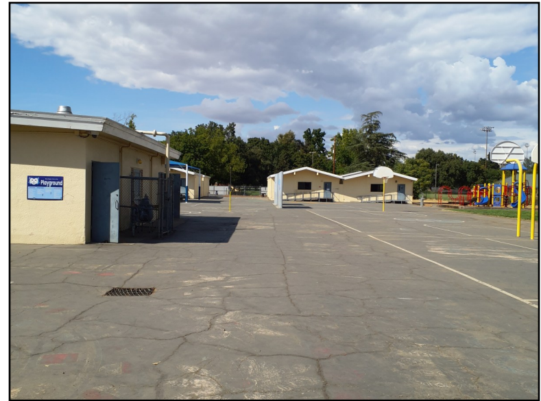
Photo 2. School Buildings (view north; September 11, 2025).
