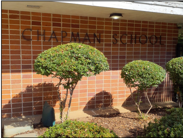
Photo 1. Chapman Elementary School Entrance (view southeast; September 11, 2025).
